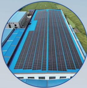
Photovoltaic Power Station Construction
